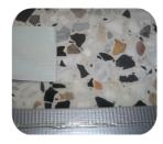
**3. Remove adhesive**To remove necessarily the adhesive bands before drying, after that will be impossible.
